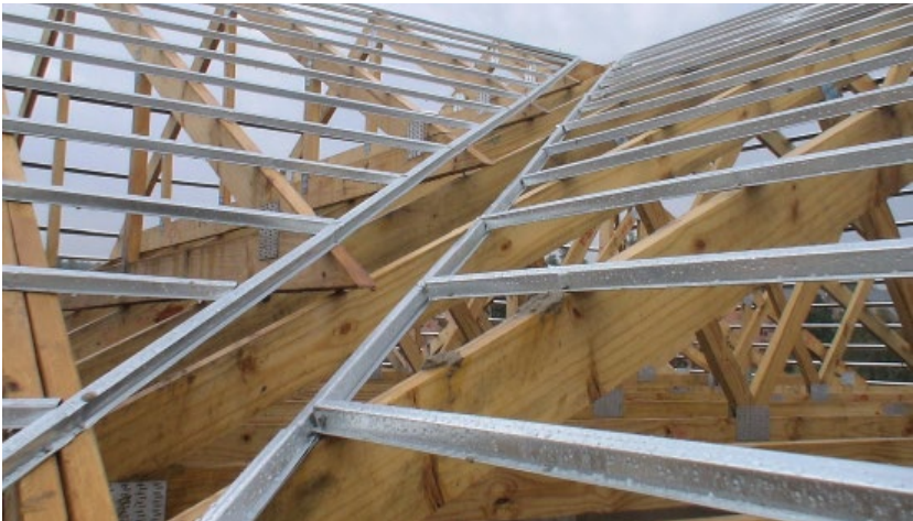
Ultra-Span® steel battens on timber trusses
