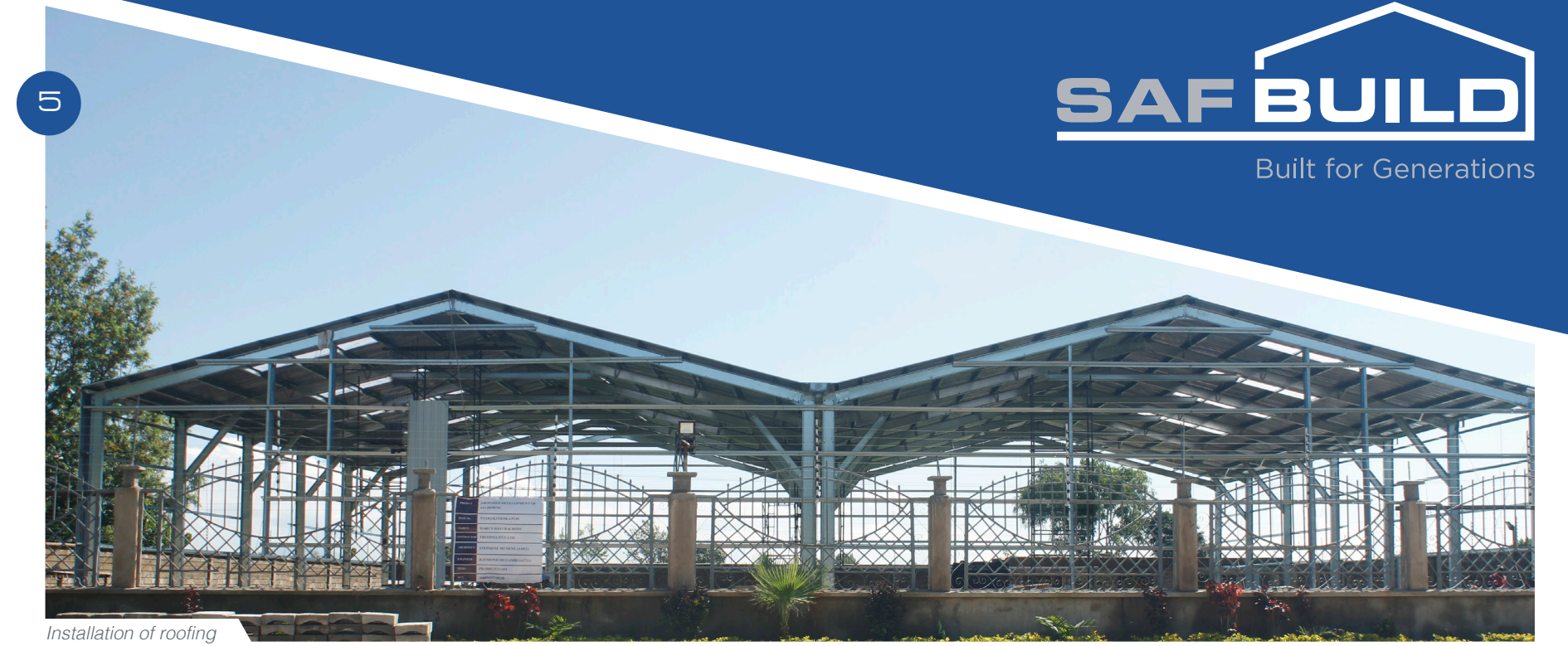
Installation of roofing
