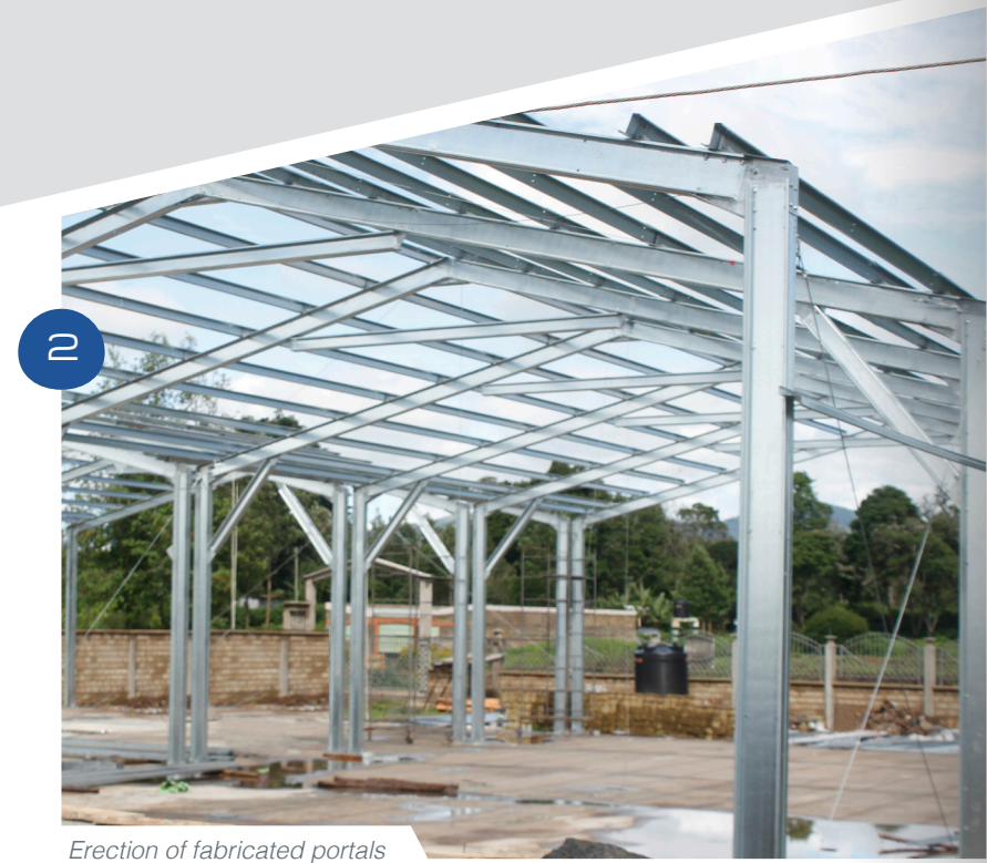
Erection of fabricated portals
