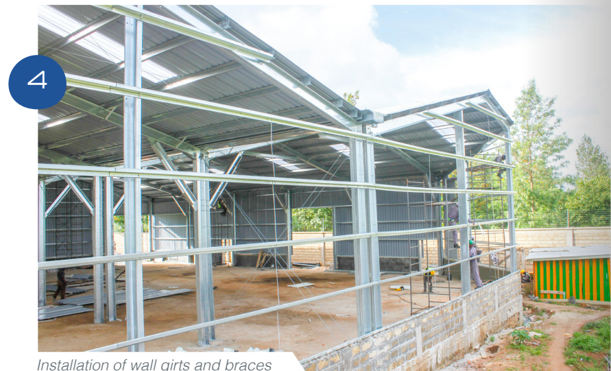
Installation of wall girts and braces
