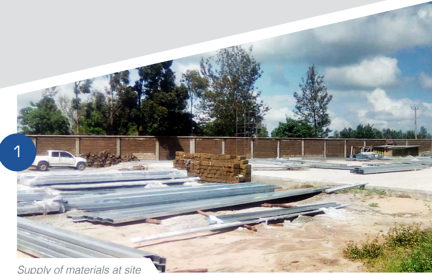
Supply of materials at site
