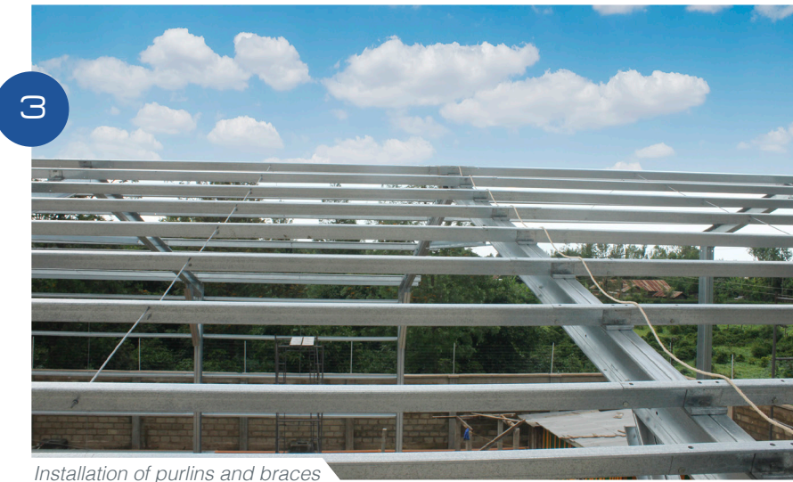
Installation of purlins and braces
