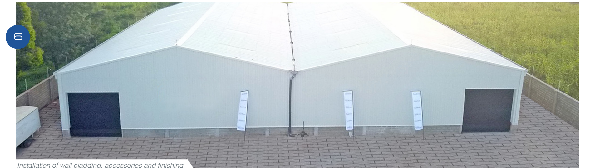
Installation of wall cladding, accessories and finishing
