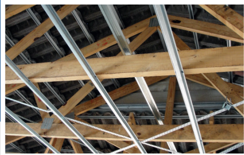
Ceiling bracing
