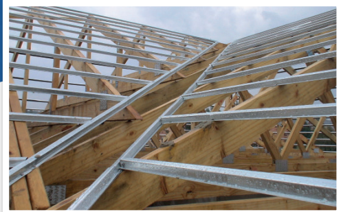
Ultra-Span® steel battens on timber trusses
